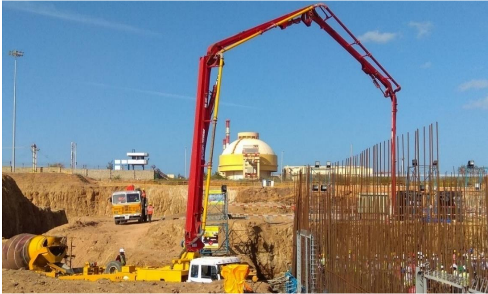
Construction at the Kudankulam Nuclear Power Plant 100
