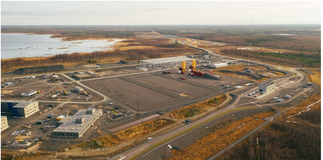
Construction site of the Hanhikivi NPP 65
